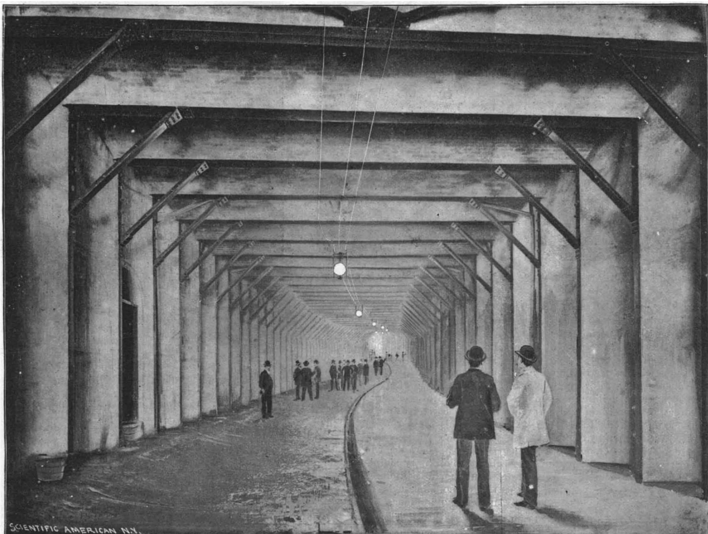
THE BOSTON SUBWAY—INTERIOR OF THE TWO-TRACK SUBWAY.
