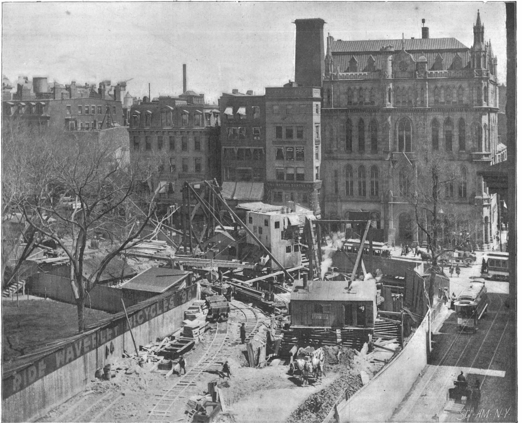
THE EXCAVATING OPERATIONS ON THE BOSTON SUBWAY NEAR THE COMMON.
