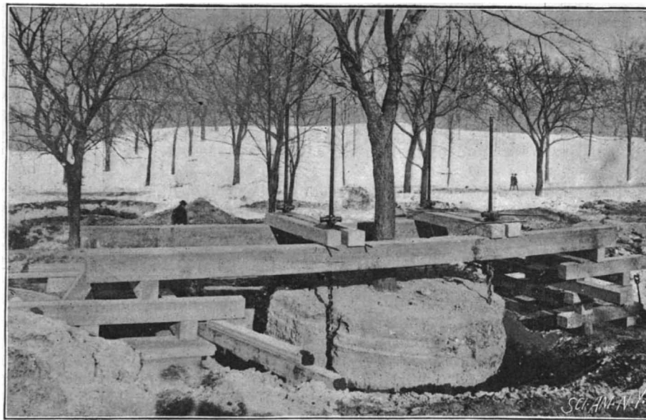
THE TREE RAISED TO ITS NEW LEVEL.
