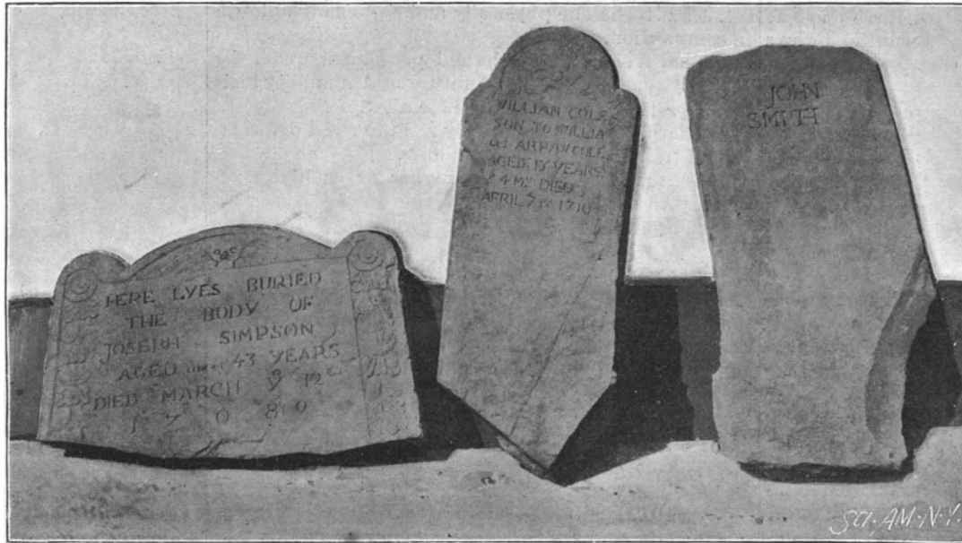
THE BOSTON SUBWAY—OLD GRAVESTONES FOUND ON LINE OF EXCAVATION.
